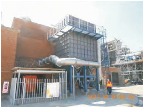
Gold Smelter High Temperature Bag Filter House
