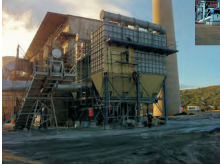
Copper Smelter High Temperature Bag Filter Houses
