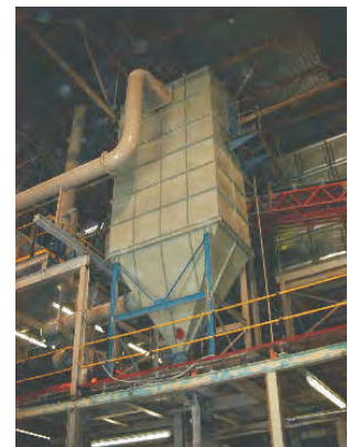
Glass Fiber Production High Temperature Bag Filter House
